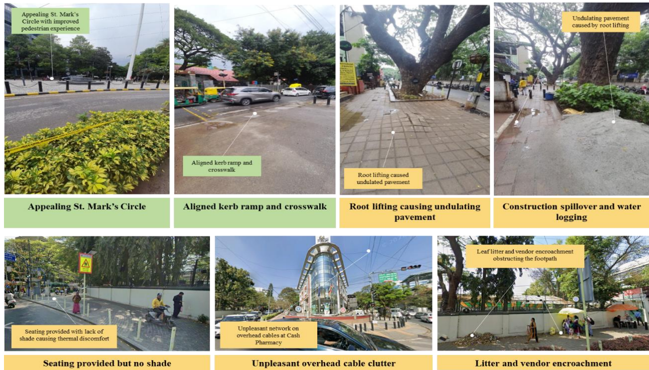
Fig. 5 Pedestrian pathway condition in St. Marks Road (Source: Author)
