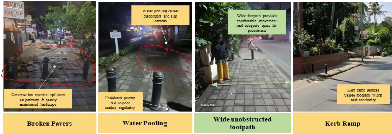
Fig. 3 Pedestrian pathway condition in Cunningham Road (Source: Author)
