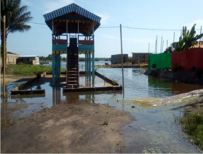
Fig. 14 Construction close to the shores in the sun district in the vicinity of the digboue lagoon
