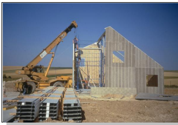
Figure 5: Erection of prefabricated cassette wall panels for house construction
