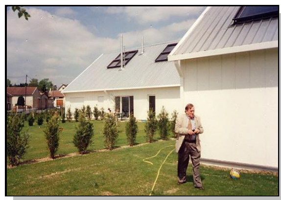
Figure 6: Houses completed with cassette wall systems
