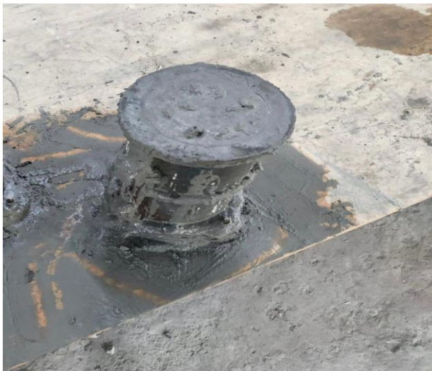
Fig. 3 Casting of cylinder specimen
