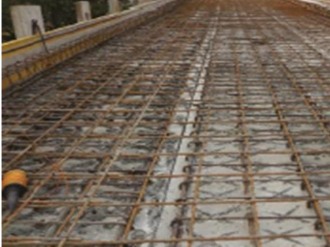
Fig. 4 Adding reinforcement for the in-situ slab
