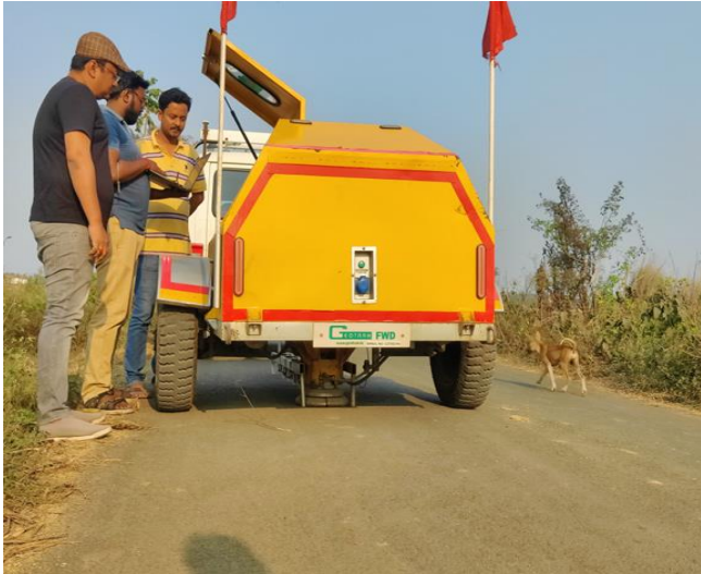
Fig. 9 FWD deflection recording on existing Jibantala-Taldi road
