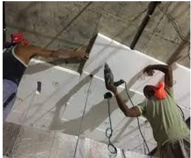
Fig. 4 Under deck thermal insulation in the building
