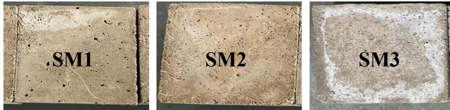
Fig. 8 Visual deterioration of samples SM1, SM2 and SM3 after exposure to sulphate attack for 180 days at 10% sulphate concentration
