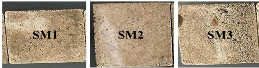
Fig. 6 Visual deterioration of samples SM1, SM2 and SM3 after exposure to sulphate attack for 90 days at 10% sulphate concentration
