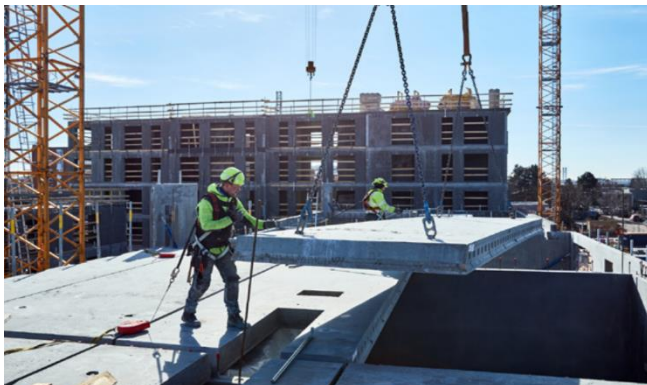
Fig. 2 Precast slab components assembly
