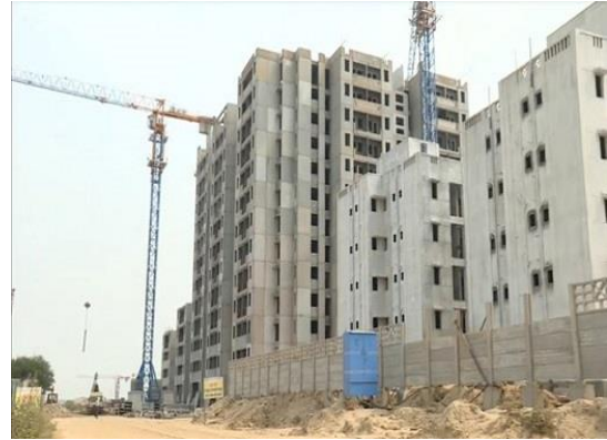
Fig. 3 Building after assembly of 3-S precast concrete construction system
