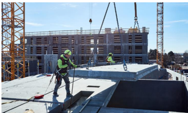
Fig. 2 Precast slab components assembly
