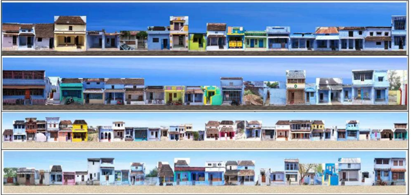
Fig. 15 Drone-captured visual documentation of building facades in Gopalamudram Agraharam Settlement
