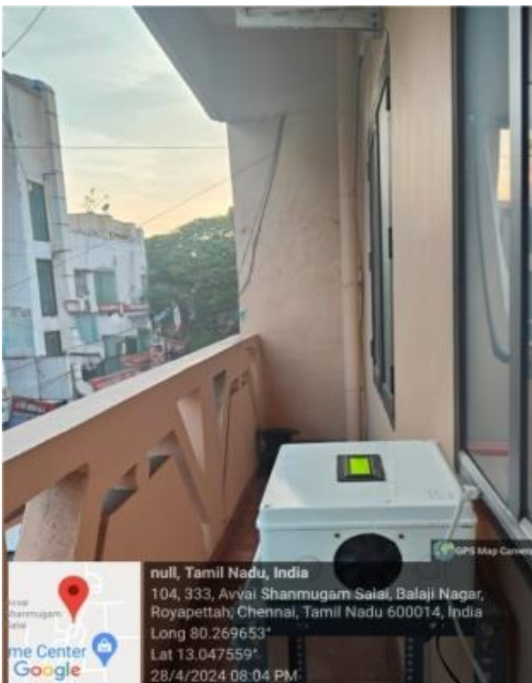
Fig. 6 An unplanted area with an Arduino controller set up
