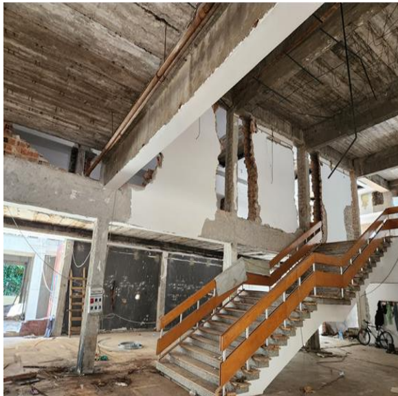
Fig. 1 Assessment of current structural conditions before intervention
