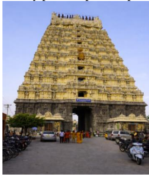
Fig. 3 Entrance gopuram - Ekambaranathar temple, Kanchipuram, Source: authors
