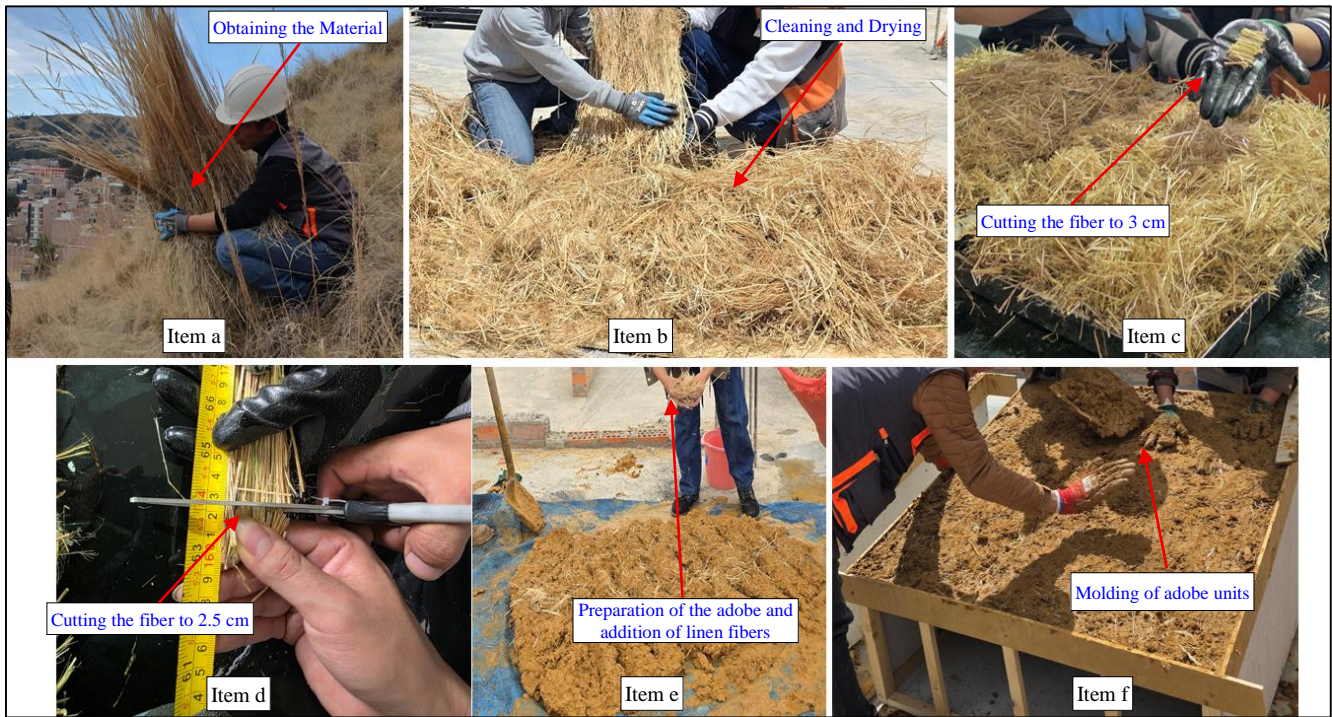
Fig. 8 Soil selection procedure for adobe with Linen
