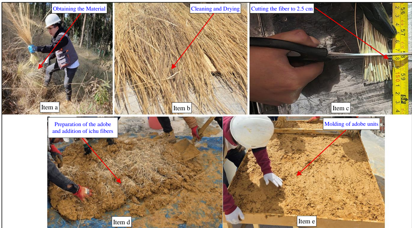
Fig. 7 Soil selection procedure for adobe with Ichu
