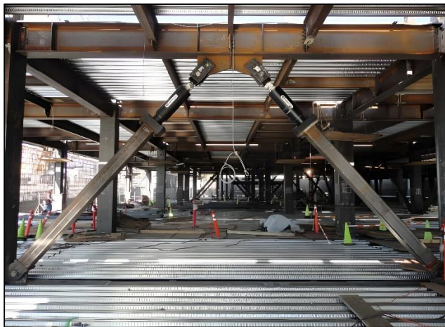
Fig. 5 Viscous fluid damper
