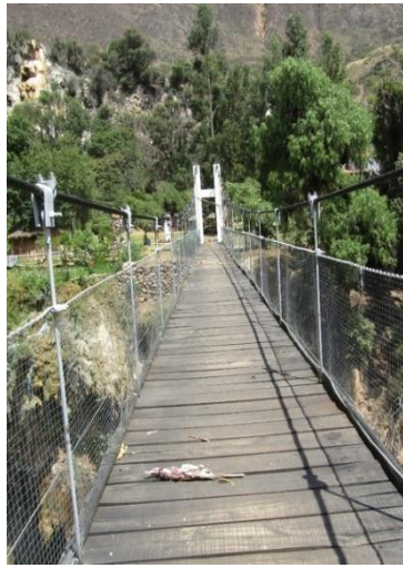
(b) Suspension Bridge 2
