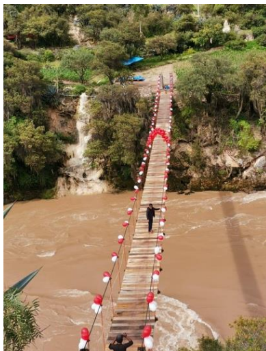
(a) Suspension Bridge 1
