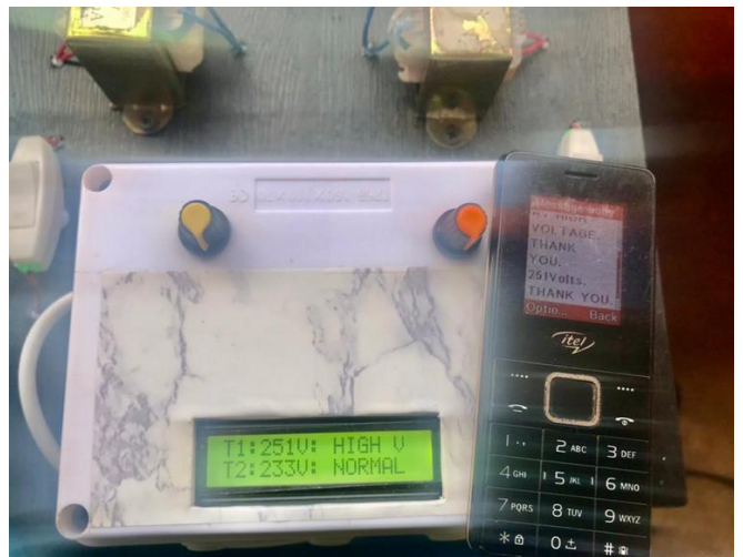
Fig. 18 The picture of the implemented system of transformer 1 at a high-voltage State
