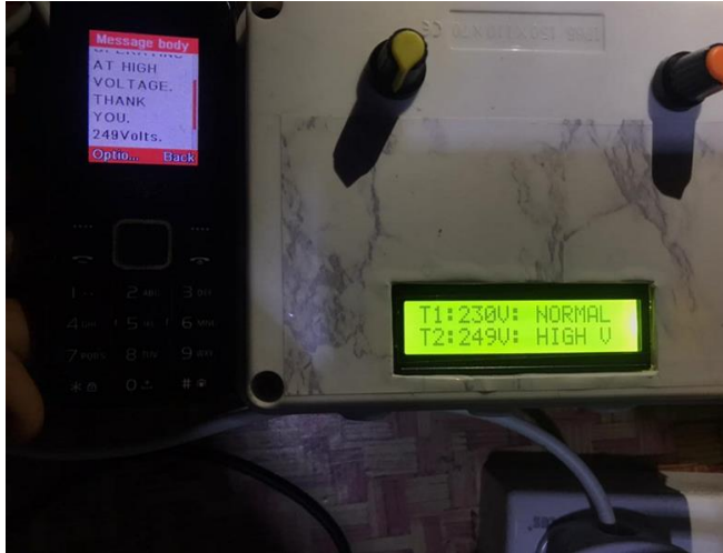
Fig. 19 The picture of the implemented system of transformer 2 at a high voltage state
