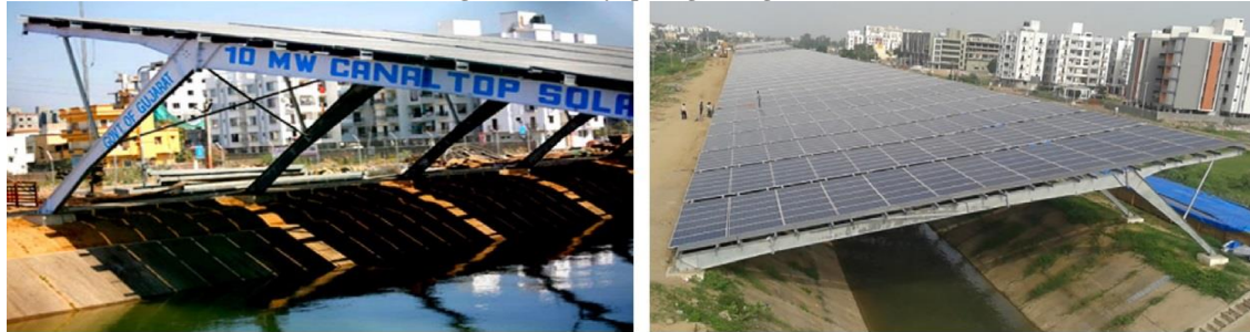
Fig. 7 Single slope due south direction arrangement
