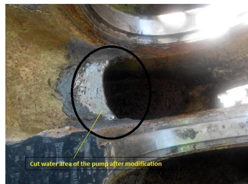
Fig-2: Cut water area of the pump after modification
